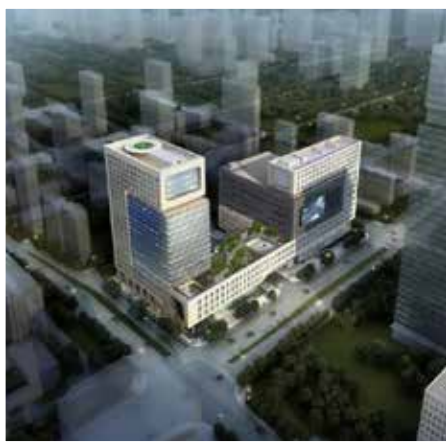
Shun Tong Building Ji'nan, China
