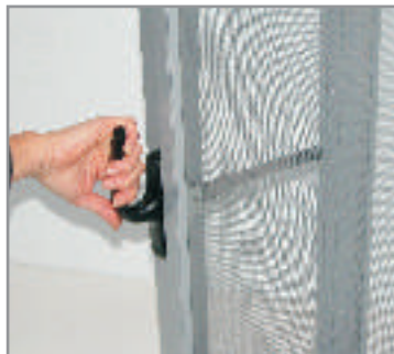
Vent attached to limit stop
