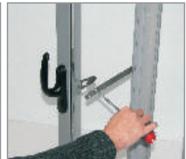
Vent disengaged from limit stop Vent fully opened
