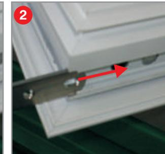
2 Fitting the arm into the groove
